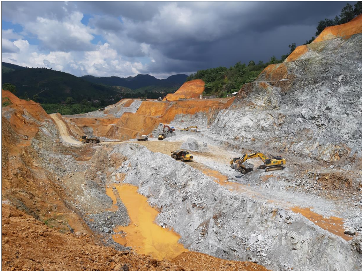
Figure 1: Talang Santo open pit looking west
