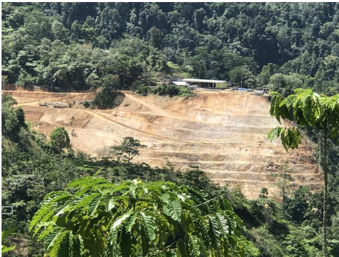
Picture 1: Open cut activities at the Way Linggo Mine
